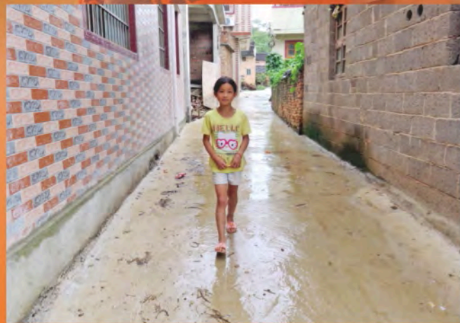
World Vision worked with community to build the concrete village road, creating a safe environment for children.
